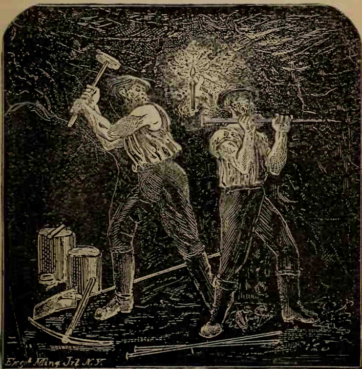
HAND DRILLING IN THE MINE.
